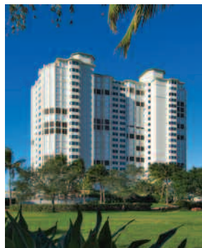
The Carlisle Naples, Florida
